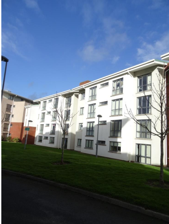
Riverwalk Student Accomodation
